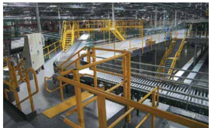
Work platforms including crossovers facilitate orderly material and safe personnel movement.
