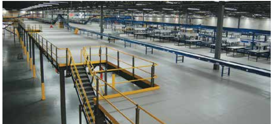
Large distribution center mezzanines maximize use of facility space.
